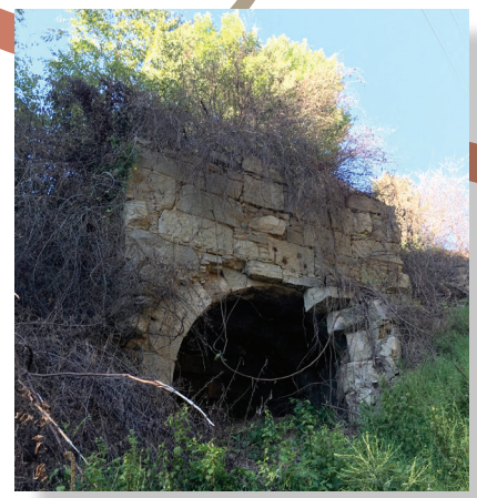
Turbine chamber ruins at Plane 5 West. Please take care exploring this site. The stonework is not maintained and may be unsafe.
